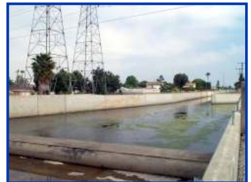
Stormwater channel with inflatable rubber dam diversion..
