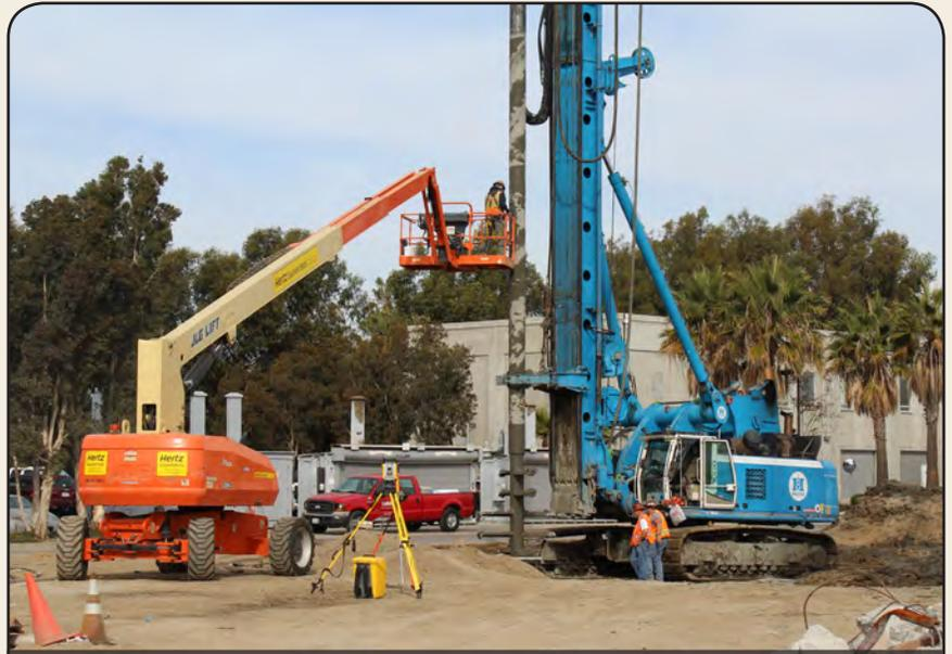
Deep soil mixing stabilizes and strengthens the soil with the use of a large auger mixing soil with cement at depths of approximately 50 feet.
